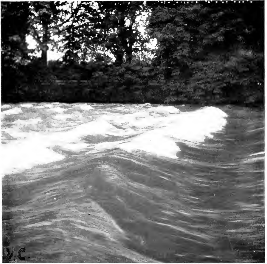
STATIONARY WAVES CAUSED BY A WEIR ON THE RIVER AARE, SWITZERLAND.
